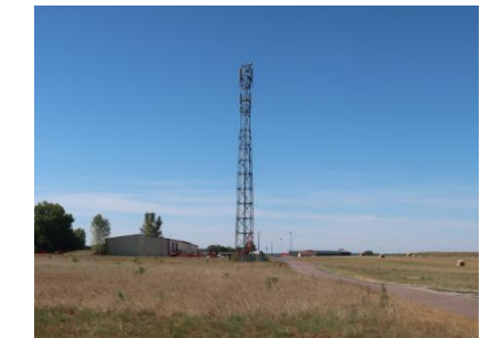
Antenne-relais Source : ARTIFEX 08/2022
