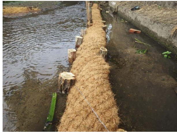
Figure 32: Principe de la Fascine
