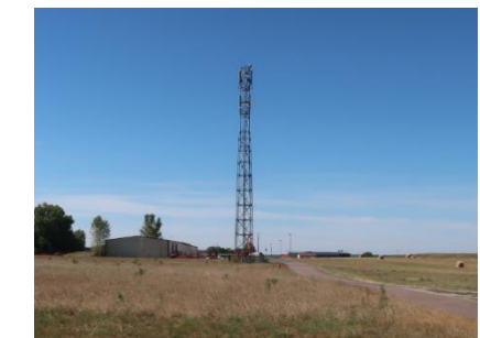
Antenne-relais Source : ARTIFEX 08/2022
