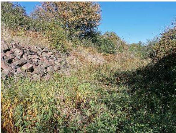
Figure 6: P3 - Exutoire trop-plein bassin C
